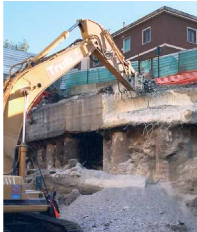
It permits a precise partial or total demolition of buildings, walkways and floors. Low vibrations transmitted to the surrounding area.
