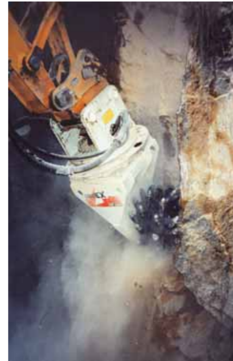
Breaking rock walls, non-invasive for the environment.
