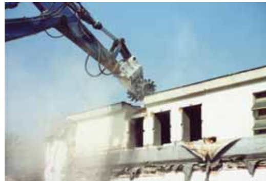
It permits a precise partial or total demolition of buildings, walkways and floors. Low vibrations transmitted to the surrounding area.
